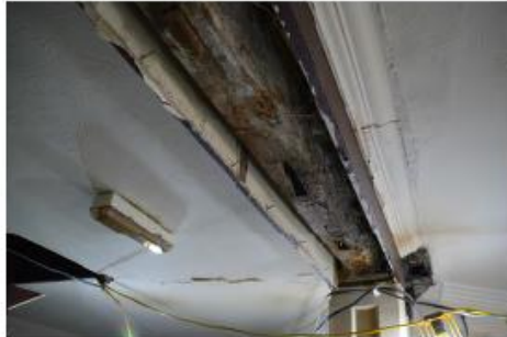
02 Opening up works. Timber casing to beam between Rooms 2 and 4 of Woodcote Cottage showing mortise evidence of a former wall.
