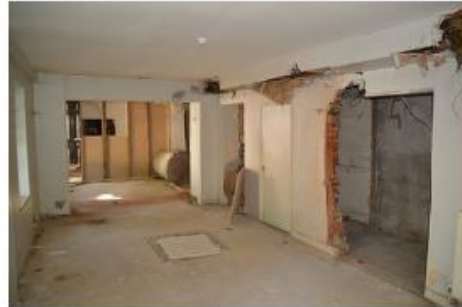
03 Unauthorised works. View inside Room 11 of Woodcote Cottage of the crudely extended opening to the original stable block.
